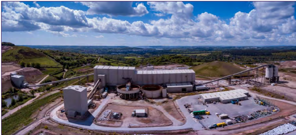
Figure 7.1 Aerial view of Hemerdon processing plant
