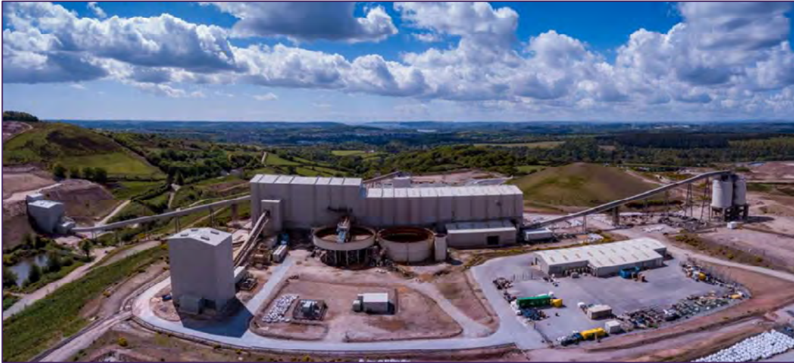
Figure ES4 Aerial view of the Hemerdon processing plant
