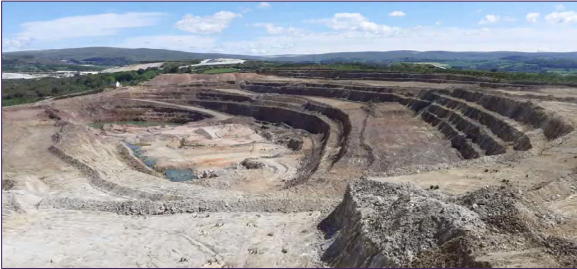
Figure 5.1 Photograph of open pit, looking north, taken on site visit (04 June 2021)
