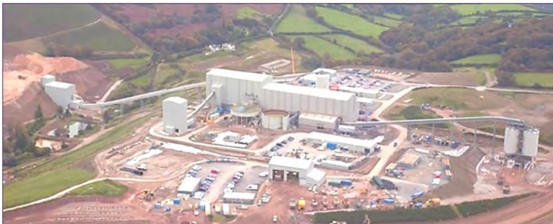
Figure 2: Aerial view of the Hemerdon processing plant (Source CPR: Figure ES4)
