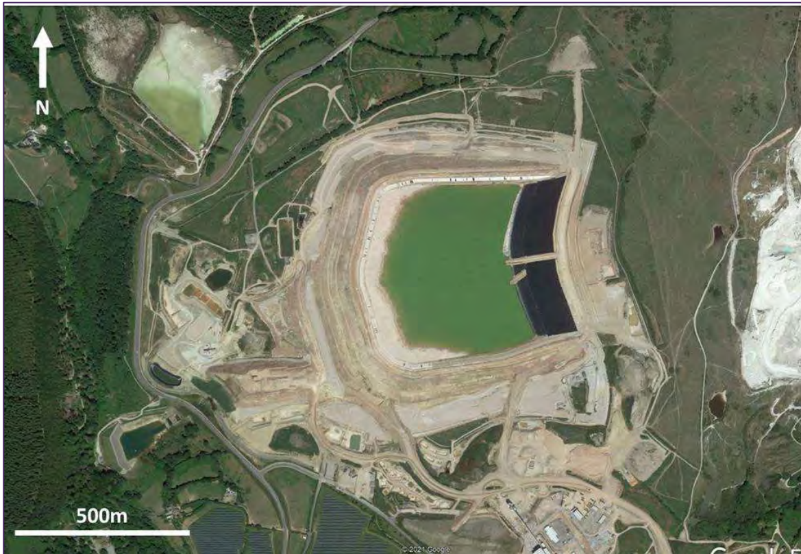
Figure 8.1 Hemerdon MWF, satellite image taken May 2020
